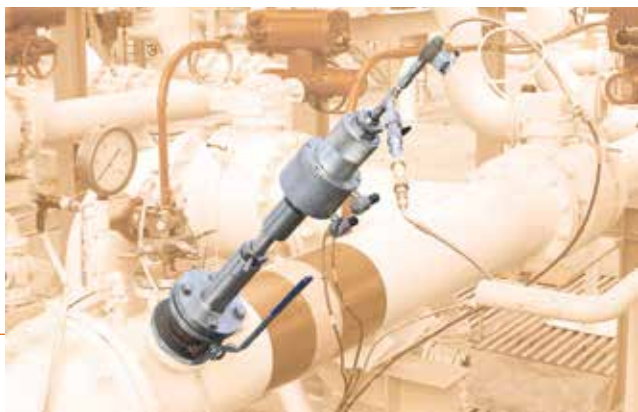
In-Line Installed probe. Sonda installata in linea.
